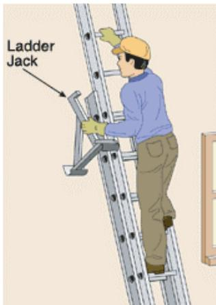
Set two ladders in position for the jacks so that when the plank is in position each of its ends will extend 1 foot beyond a jack. If using a 10-foot long plank this means setting the ladders about 8 feet apart. Check that each ladder is level and stable. Working one ladder at a time, carry up a ladder jack and, at the desired height, secure the jack properly to the rung. Make sure that both jacks are set to an equal height.
